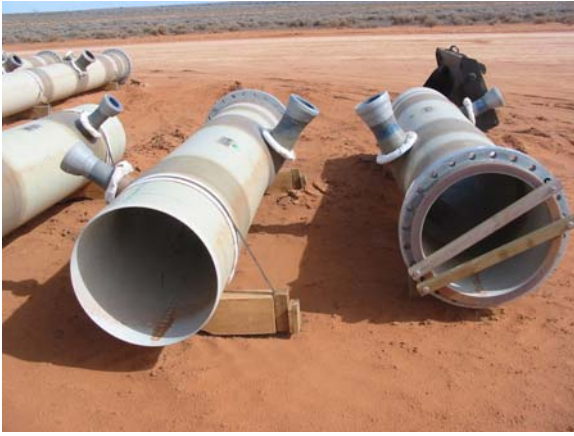
Figure 2: GRP monolithic pipe “specials” serving as isolation valve assemblies. Each fitting contains a scour and air valve tee, one flanged end and one scipgot end.
