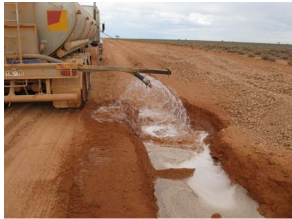
Figure 1: Conditioning of trench backfill with untreated groundwater from the J-A borefield.
