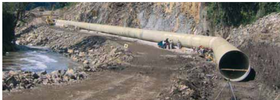
Amiantit (Saudi Arabia) is able to produce pipe that is four meters in diameter with highly robust flexible joints for high pressure applications.
